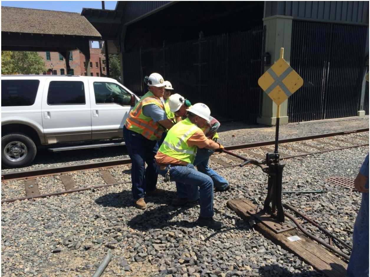
The Carlson Tool is deployed. Chris, Steve, and Ed use the proper tool for straightening the stand
