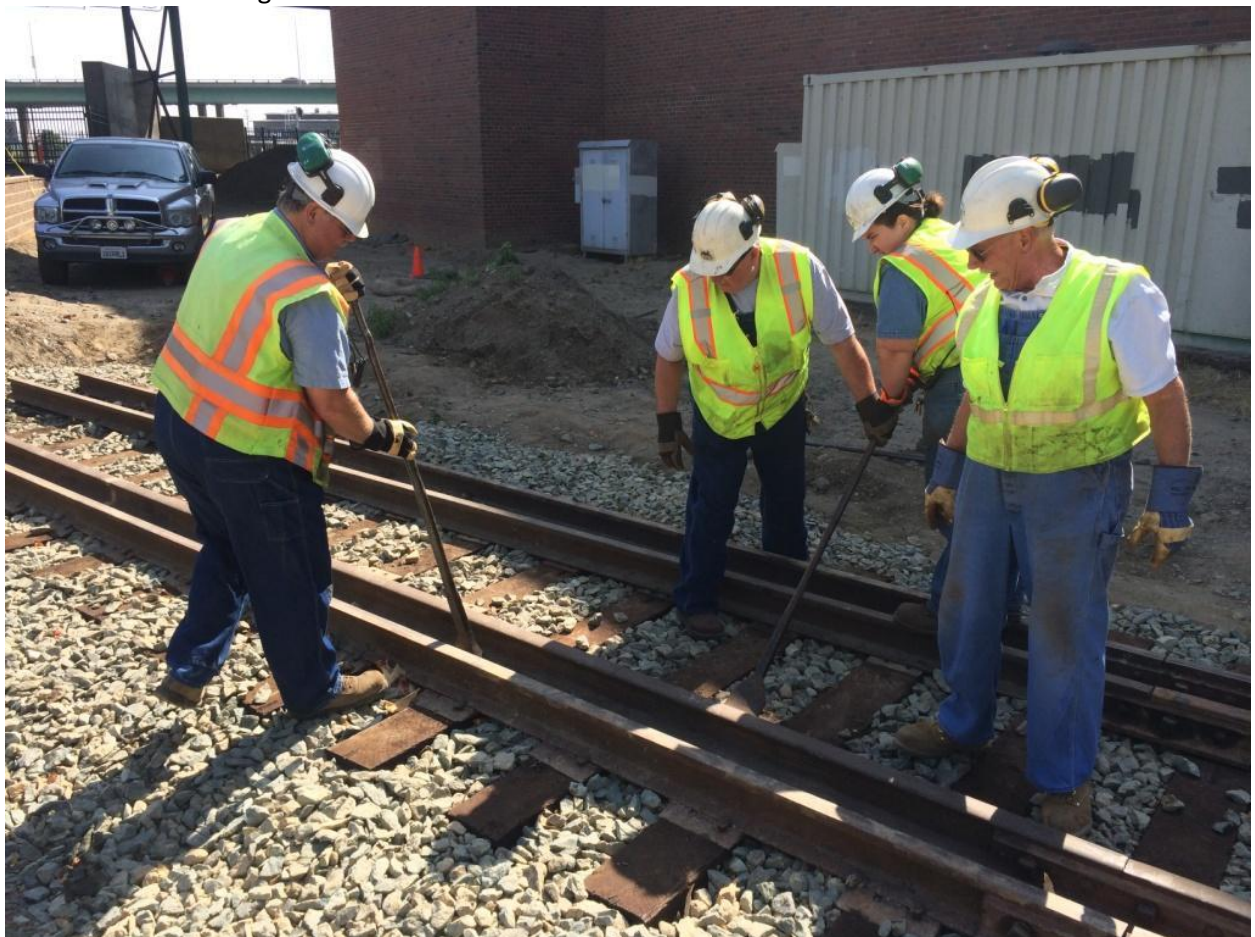
Chris, Harry, Heather, and Clem nip the west rail of west narrow-gauge track
