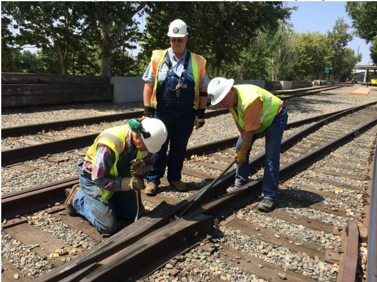
While on the scene, Steve, Chris, and Ed tighten a hard to access bolt in the frog at Switch 5
