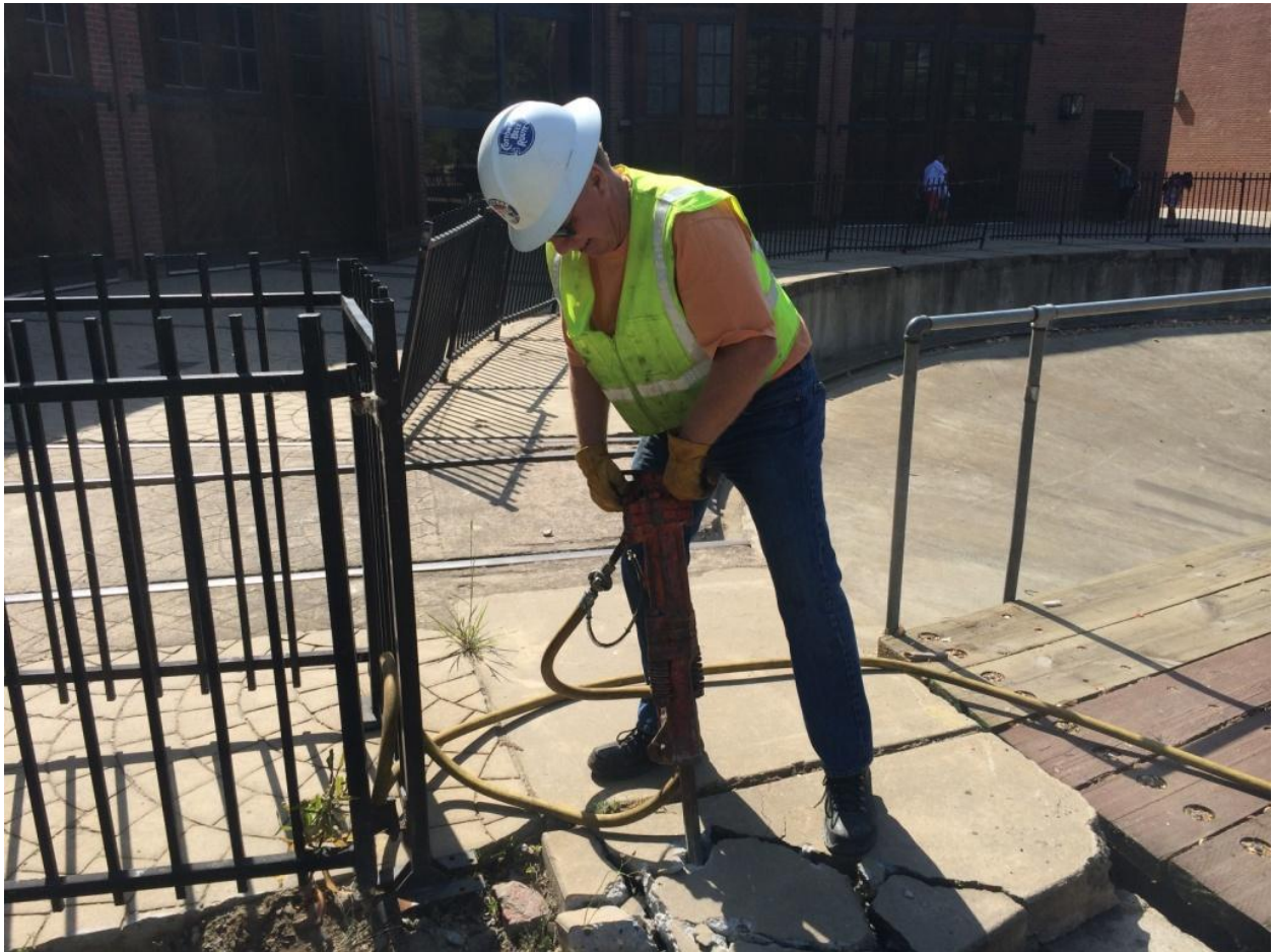
Ed jack-hammers the apron around the turn-table in preparation for the new fence
