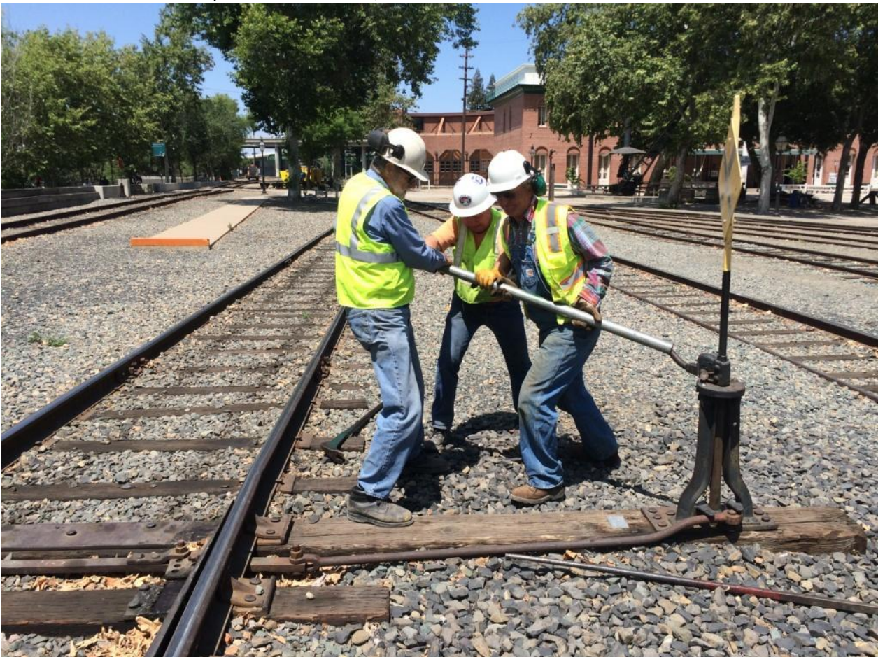
Alan, Ed, and Steve making the first attempt at straightening the switch stand
